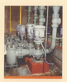
PROCESS SYSTEM: Horizontal split case pumps provide process cooling water for this major customer. Energy efficient operation and mechanical reliability were major considerations for this critical application.
